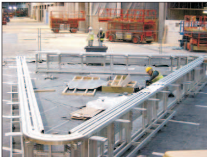
Start of an installation in a new shopping centre
